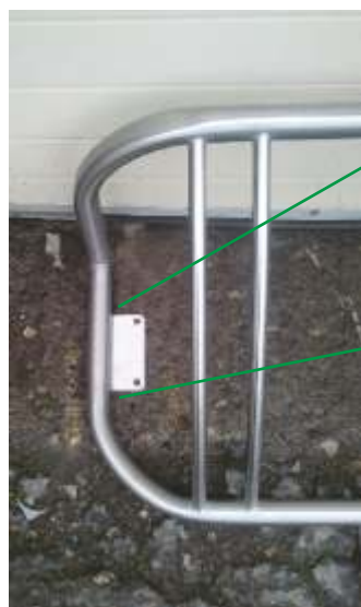
Baseplate fixing detail for cycle stand
