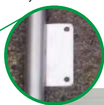
Baseplate fixing detail for cycle stand
